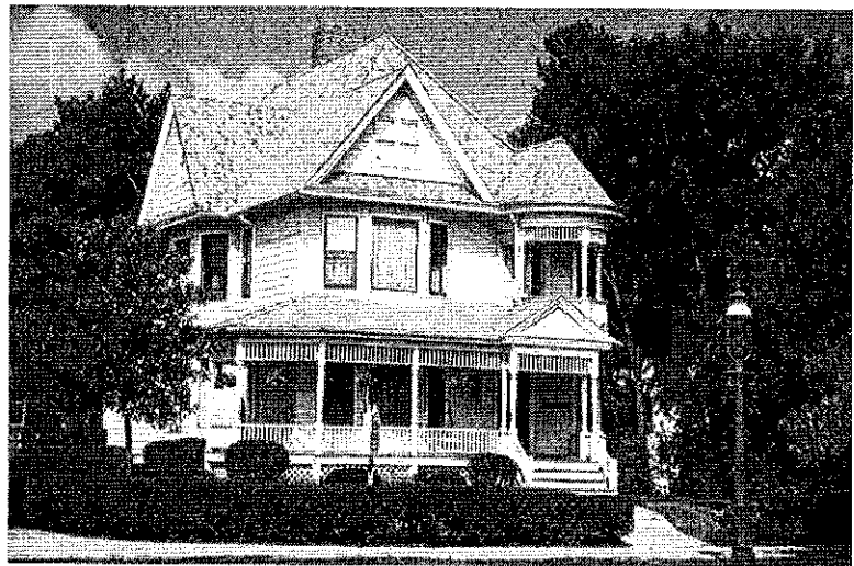
FIGURE 3. This house has been framed with trees.
